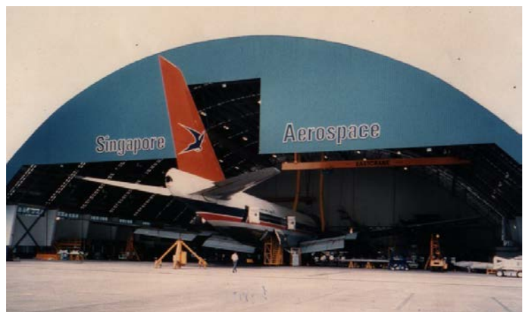
Fig. 5 Completed SAE Hangar
