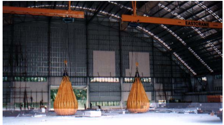
Fig. 6 Proof Testing of Cranes in SAE Hangar
