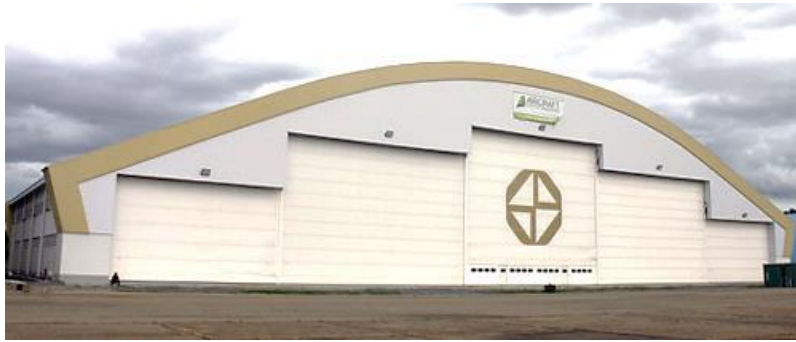
Hangar Exterior completion in August 2016
