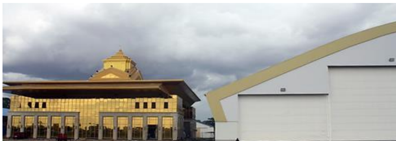
Business Jet – Fixed Base of Operations (FBO) Exterior
